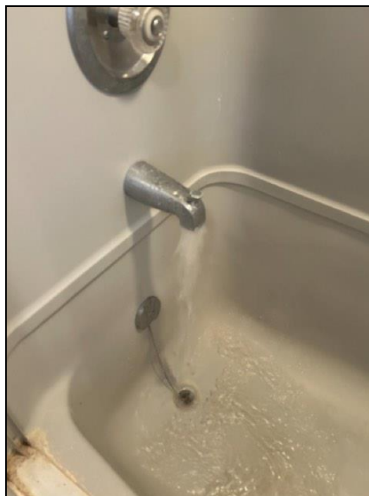
71. All plumbing tested inside home. Water let...
