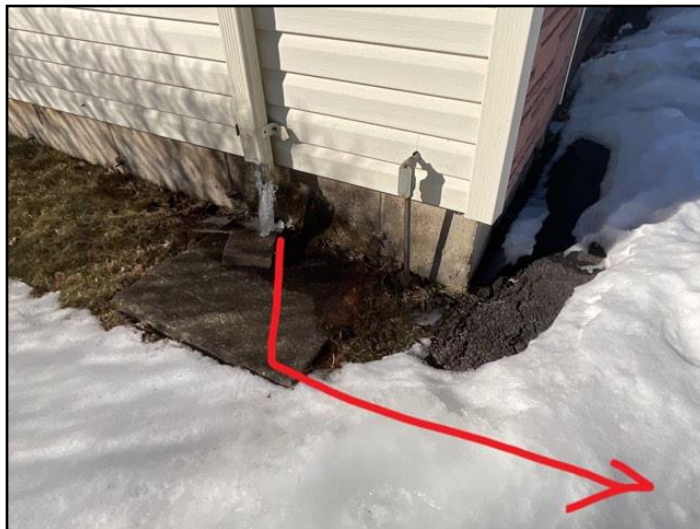
8. Add downspout extensions to get water away...
