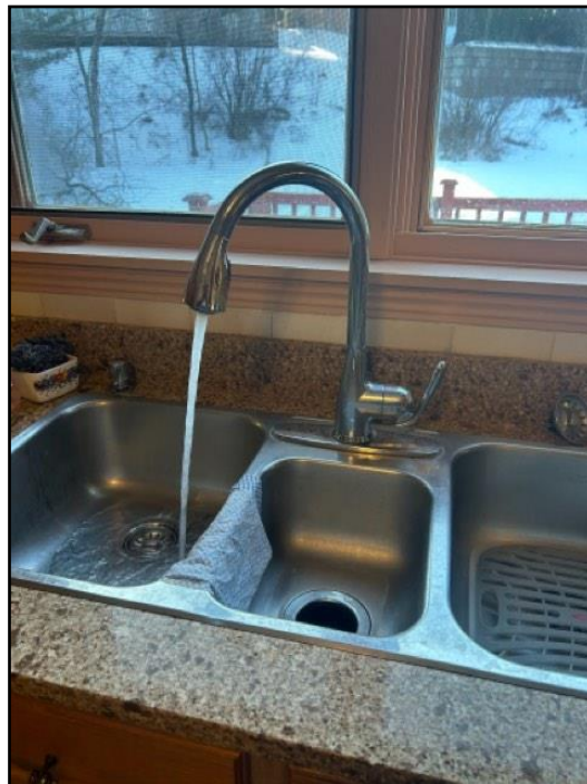
77. All plumbing tested inside home. Water let...
