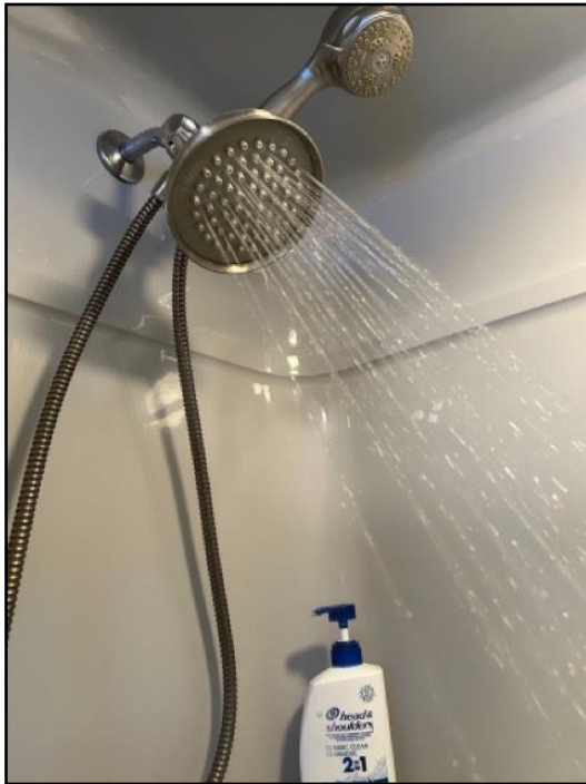
72. All plumbing tested inside home. Water let...
