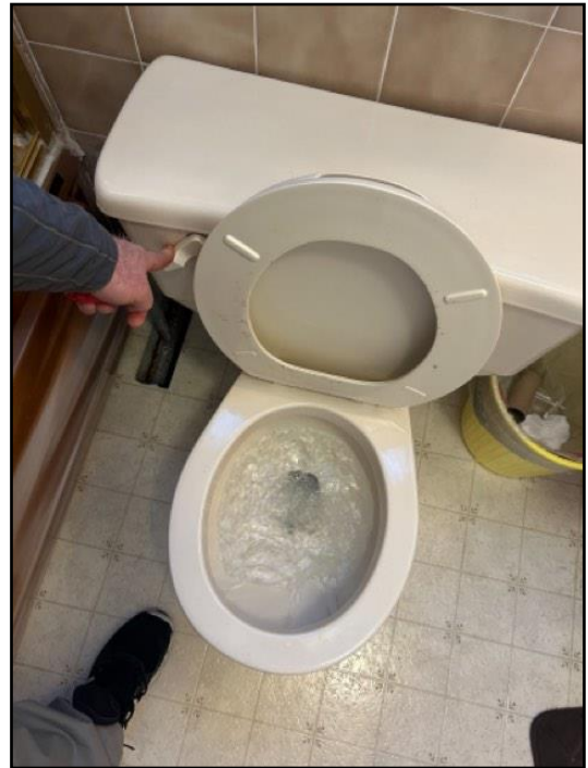
73. All plumbing tested inside home. Water let...
