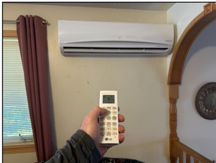
62. Ductless (Mini split) system
