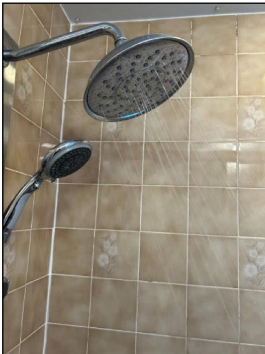
74. All plumbing tested inside home. Water let...
